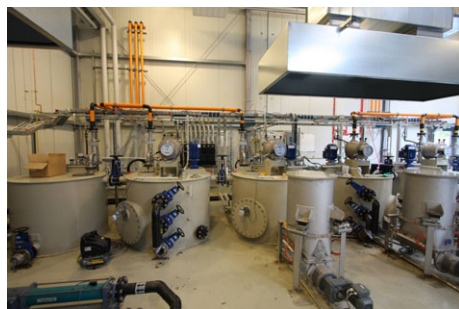
Figure 3. Pilot-scale plant used for testing.
